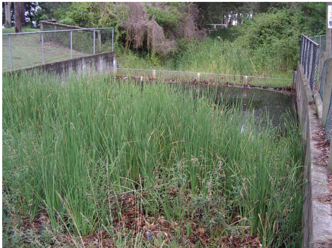
Figure 21. Artificial wetland and gross pollution trap.
