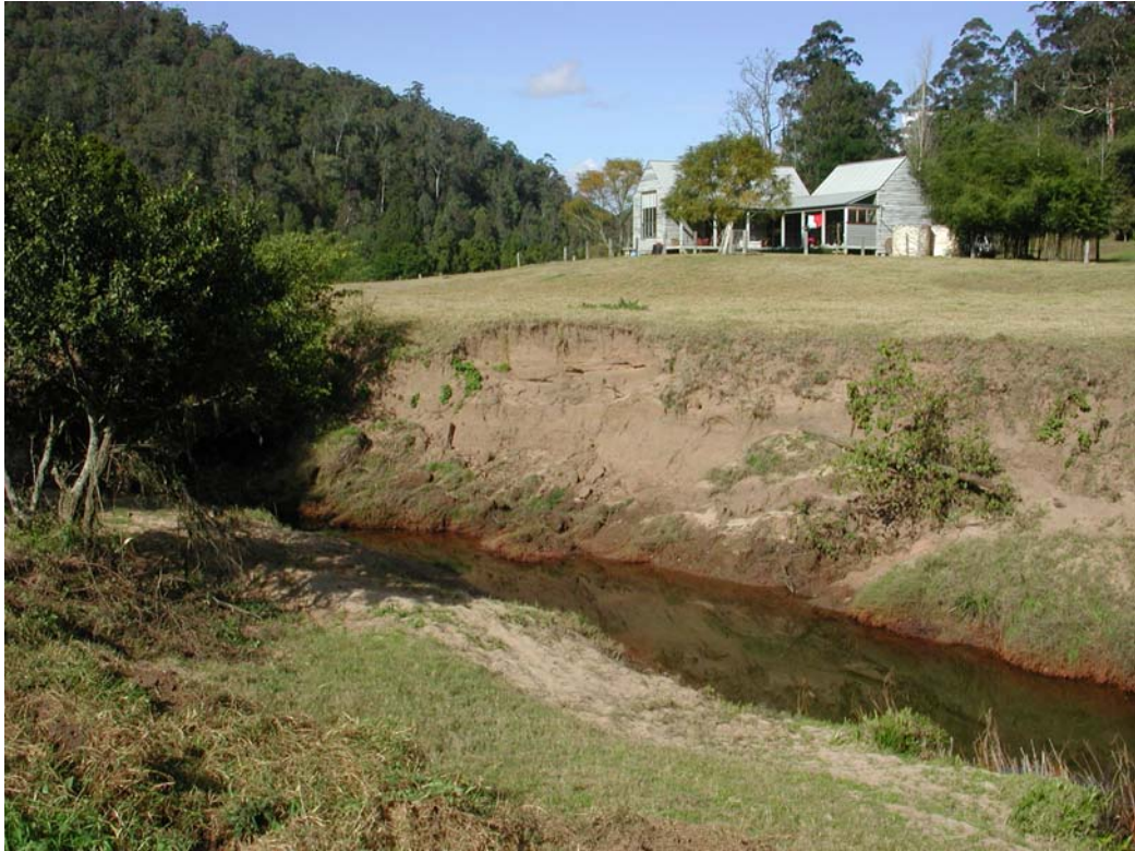
Figure 22. Streambank erosion before rehabilitation.
