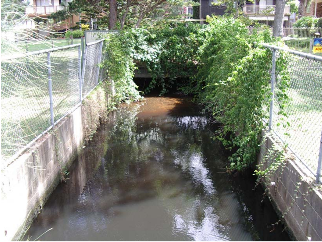
Figure 20. Stormwater drain entering the lake.
