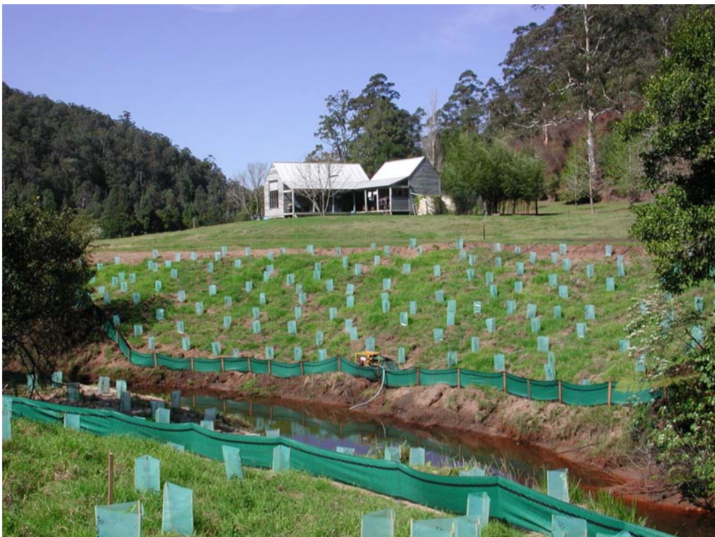
Figure 23. Streambank after rehabilitation.
